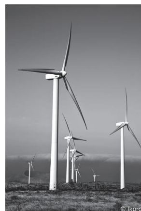
Fig. 4.16 Wind turbines on a wind farm. Wind power creates no emissions and is reasonably efficient
